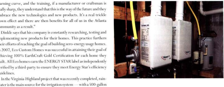
this system heats water on-demand and delivers an endless supply of hot water for as long as the homeowner needs it.
